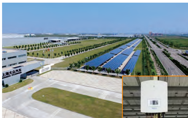
Shanghai Volkswagen Photovoltaic solar carport 55MW
