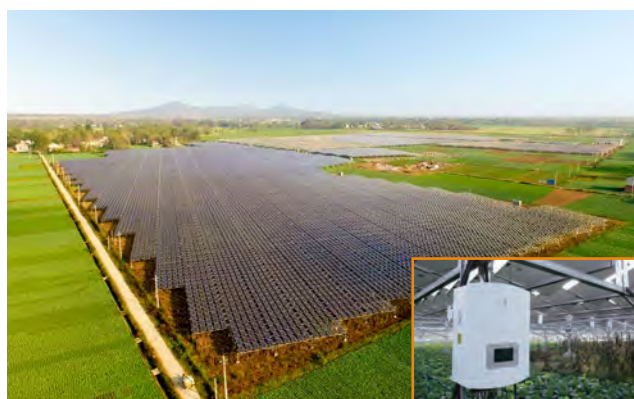
Hubei Guanyin Agricultural-photovoltaic hybrid PV plant 20MW
