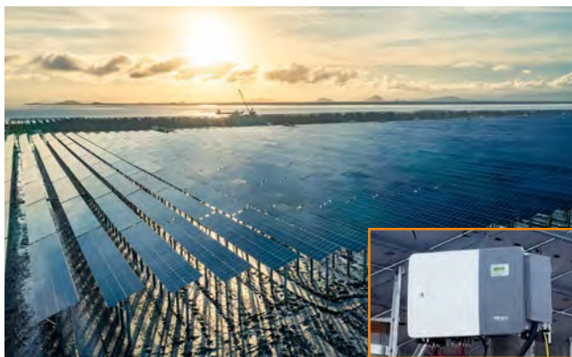
Zhejiang Ningbo Tidal Flat Project 300MW
