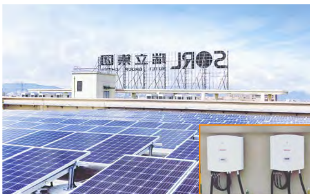
Zhejiang SORJ 3.9MW
