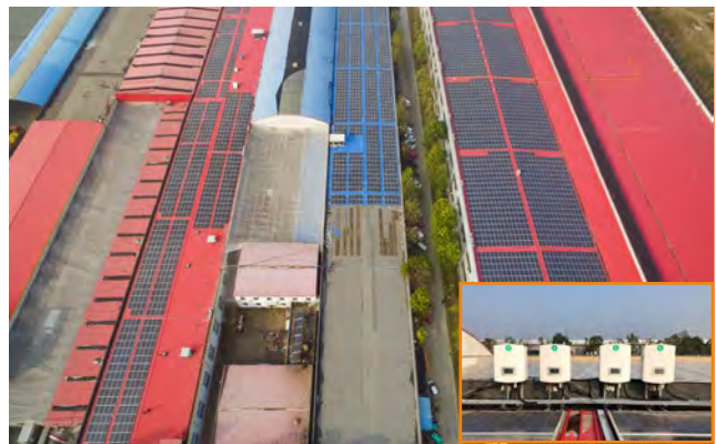
Shandong Weifang Linqupoverty alleviation PV Plant 20MW
