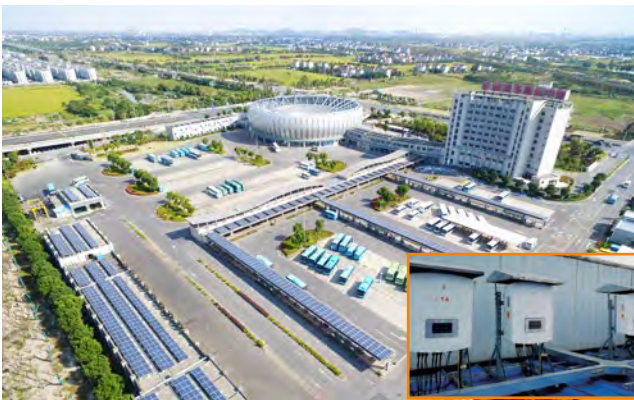
Zhejiang PINGHU Bus Station 472kW
