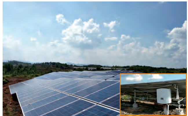
Jiangxi Ganzhou PV Plant 3.5MW
