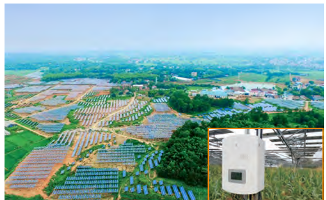
Quzhou Qinghu Agricultural-photovoltaic hybrid PV plant 20MW
