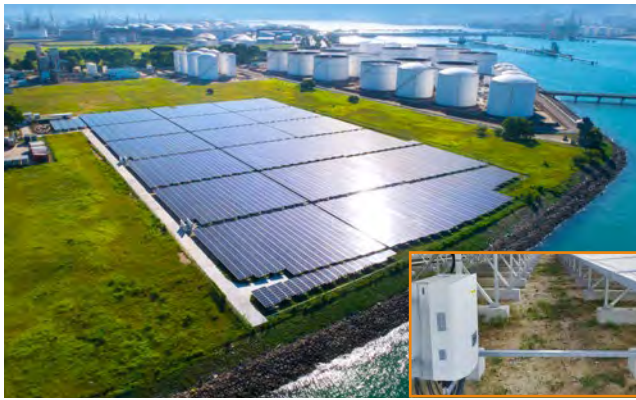
JTC Solar Farm, Singapore 5MW
