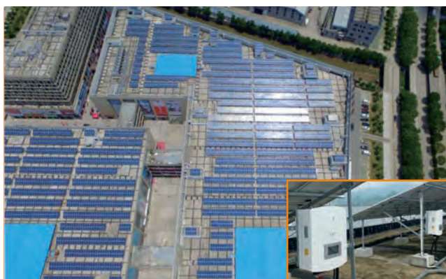
Ninghai AB hall, modern home plaza 1.53MW
