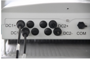
▲ Figure 4.9 Connect the DC Connectors to the Inverter
