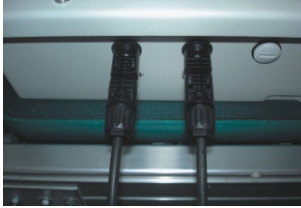
▲ Figure 4.9 Connect the DC Connectors to the Inverter
